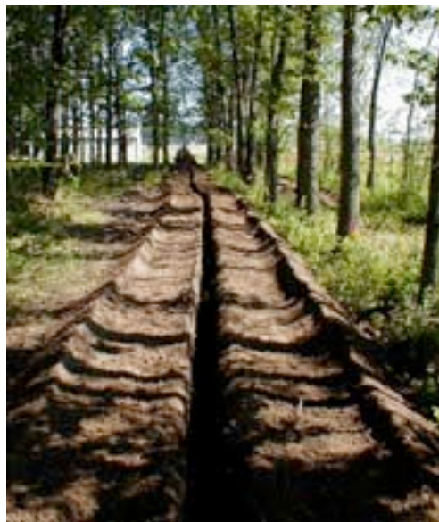
Figure 1. Trenches, dug with a Davis Fleetline 70+4 trencher, were used to isolate treatment groups.
