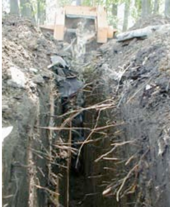
Figure 2. Five to six-foot-deep (1.5-1.8 m) trenches break potential root grafts between neighboring trees. Trenches are approximately 4-6 in. (10-15 cm) wide.
